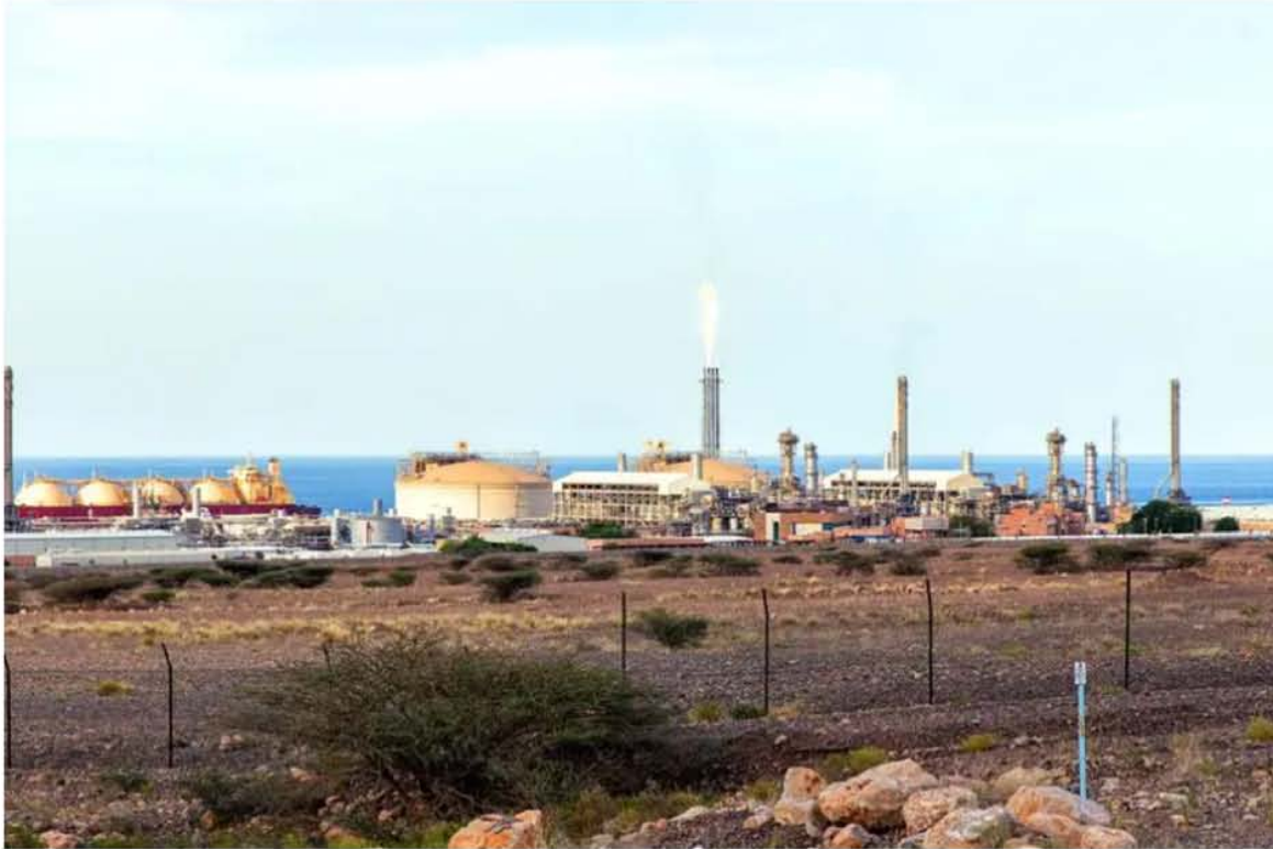
Desalination plant on the seashore in the city of Sur, Sultanate of Oman. Getty Images Image used for illustrative purpose. Getty Images
